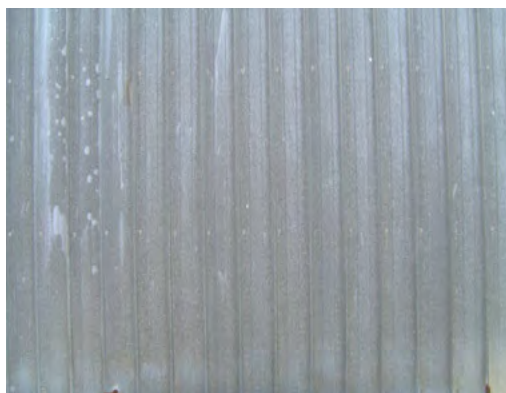
Galvanised panels used for walls or roofs.
