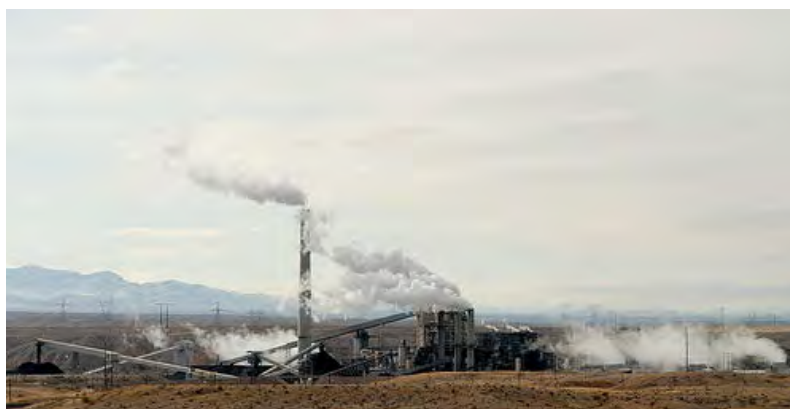
A coal-powered power station.
