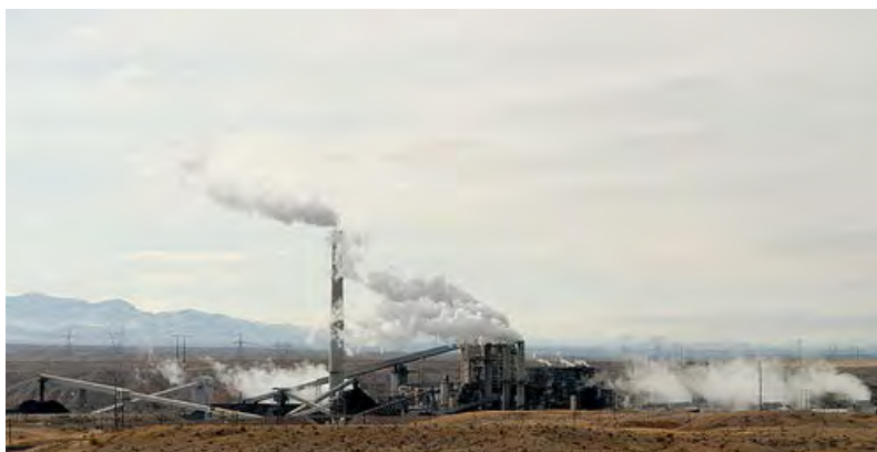
A coal-powered power station.
