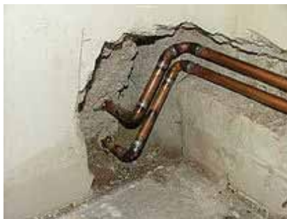
soldered copper pipes
