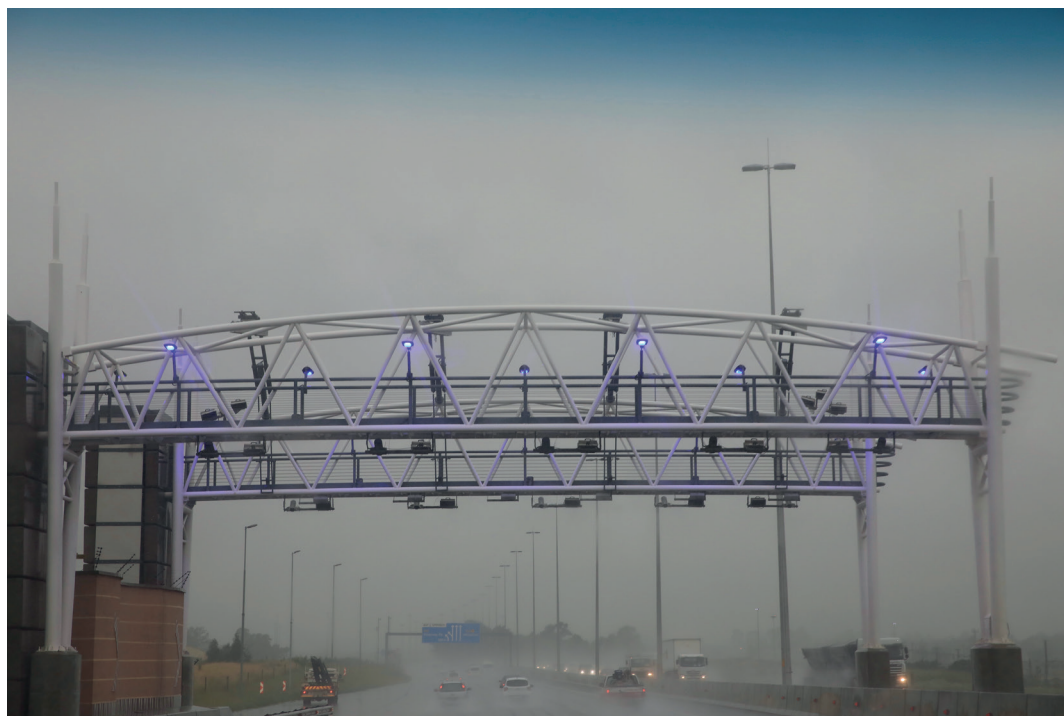
Figure 1.2: An e-toll gantry
