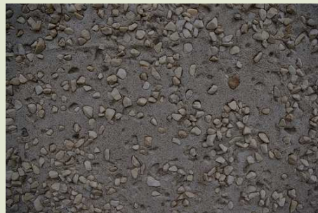
A close up photo of a slab of concrete. 5
