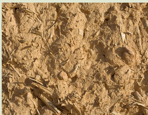
A close up photograph of a mud used to make the wall.
