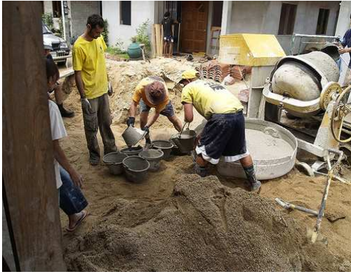
Mixing cement using a mixer.
