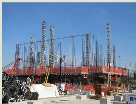
A new building. 7
