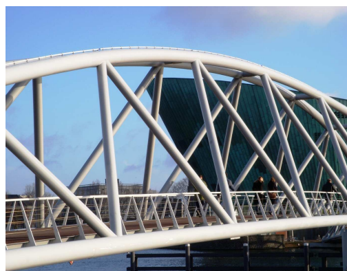
A bridge made of metal.
