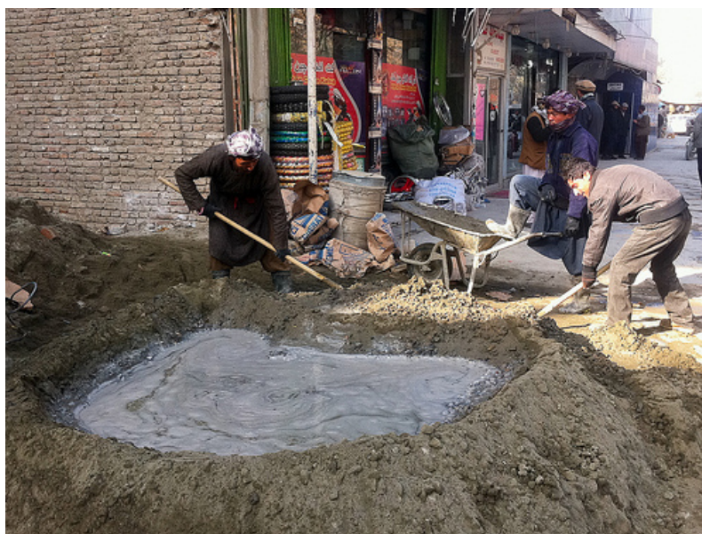
Mixing cement using spades.
