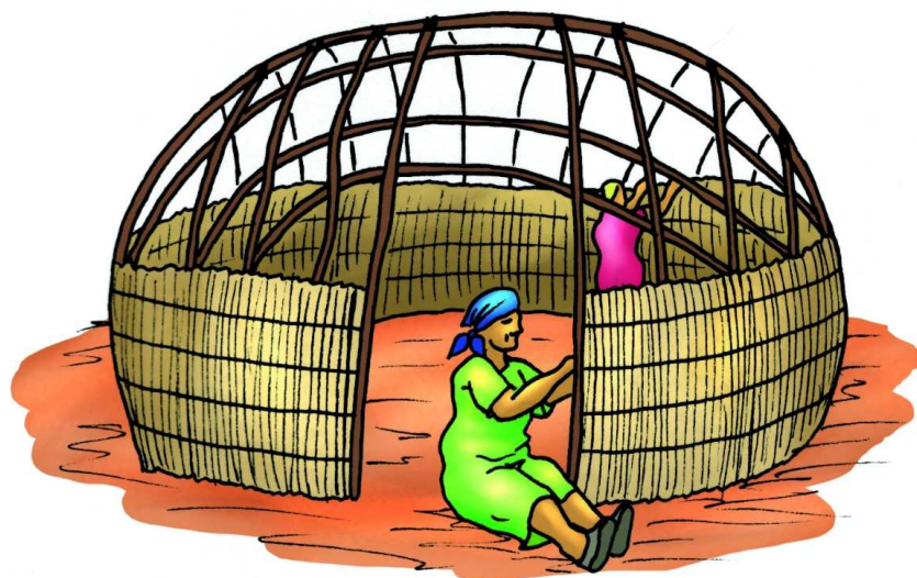
Women attaching the reed mats to the framework.
