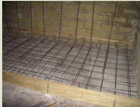
A piece of floor being prepared. 6
