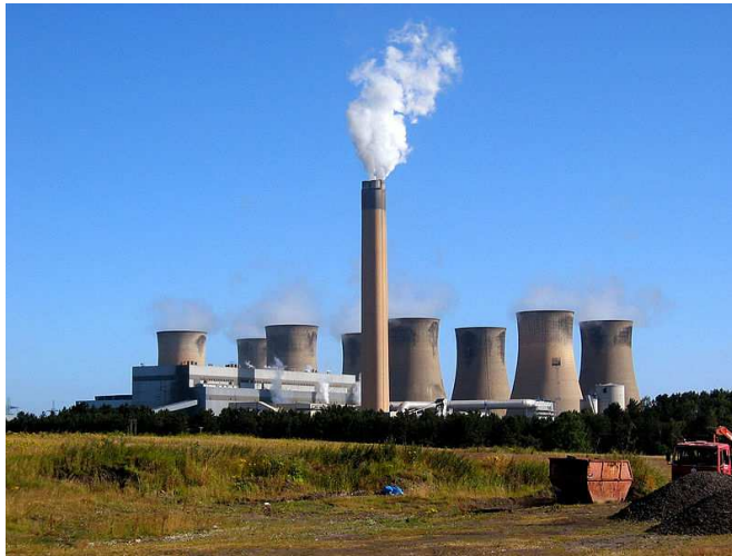
A power station
