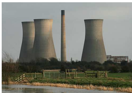
A power station 4
