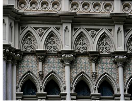
Decorative carvings and columns made from sandstone on the front of a building 13
