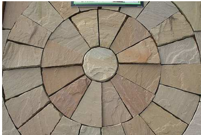
Paving blocks made from sandstone 14
