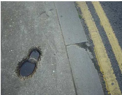
A footprint which has hardened in the cement 7
