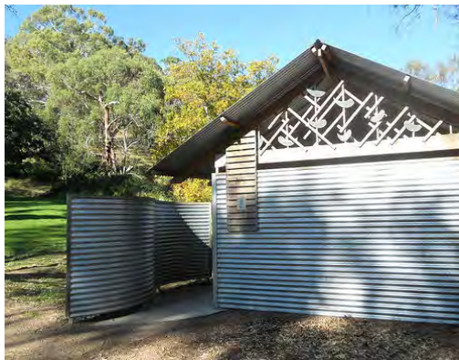
The walls and roof of this house are made of sheets of corrugated metal.
