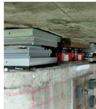
Figure 5.9d There is a bearing between each of these supporting columns and the bridge structure above.
