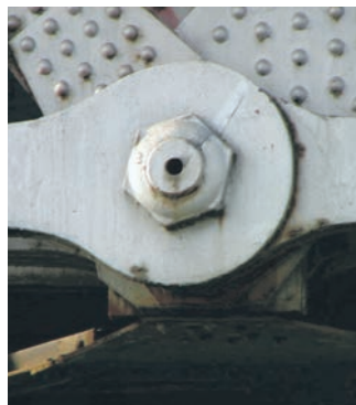
Figure 5.9a A pinned joint
