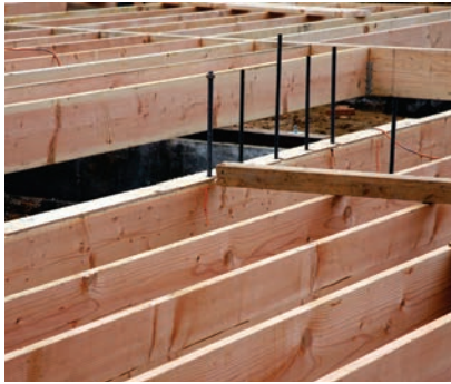
Figure 3.24a Wooden floor joists
