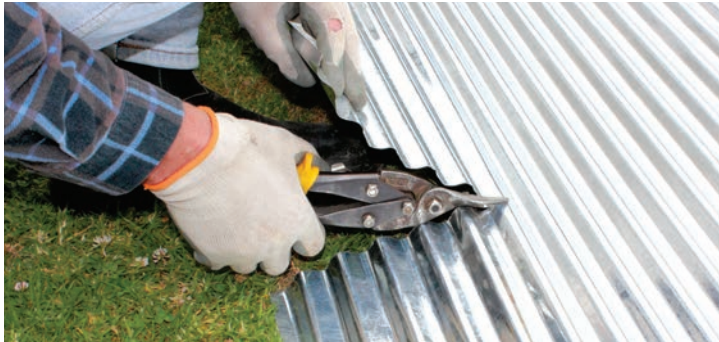
Figure 3.25 Tin snips cut the sheet metal with a shearing action.
