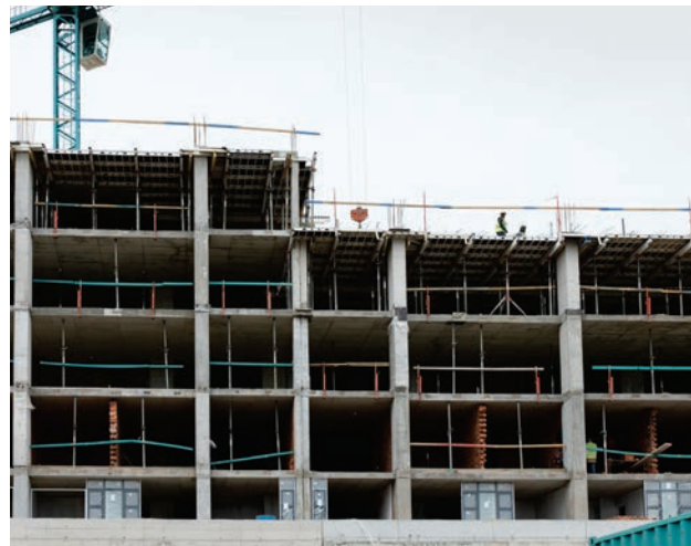
Figure 3.20b Columns of a concrete framed building
