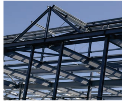
Figure 3.24c Steel beams in a steel-framed building
