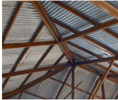
Figure 3.24b Wood purlins that support a “corrugated iron” roof
