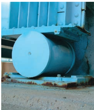
Figure 5.9d There is a bearing between each of these supporting columns and the bridge structure above.
