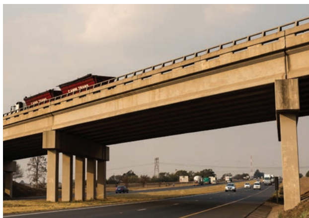
Figure 5.10a Simply supported beams in a bridge
