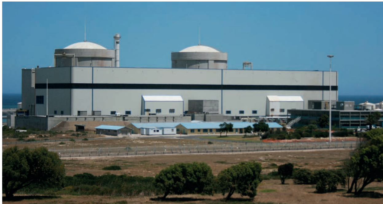
Figure 8: A nuclear power station
