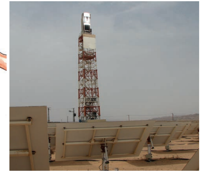
Figure 10: Thousands of mirrors at a solar thermal power station all reflect sunlight onto a tank on top of a tower. That is why the tank is shining so brightly.
