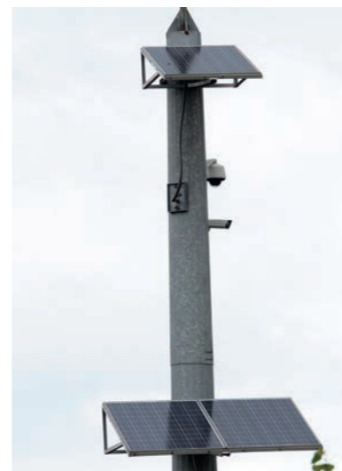
Figure 14: Photovoltaic cells on a pole
