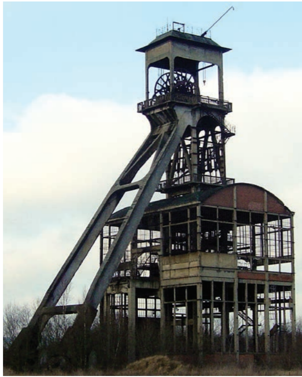
Figure 1: This is the tower above an old mine shaft. A cable winds around “sheave” wheels on the “headgear” at the top. These cables are attached to a lift that transports miners, machines and ore into and out of the mine.
