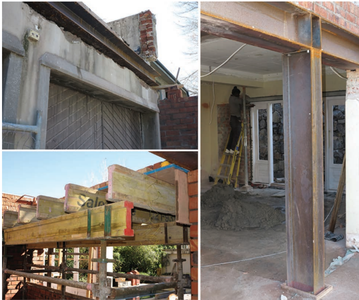
Figure 25: Steel I-beams are often used in buildings. Wood I-beams are often used during the construction of a building, but are removed once the building can support its own weight.
