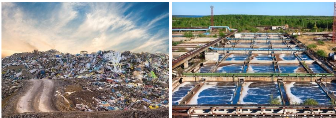
Figure 7: Solid waste disposal and water treatment plant
