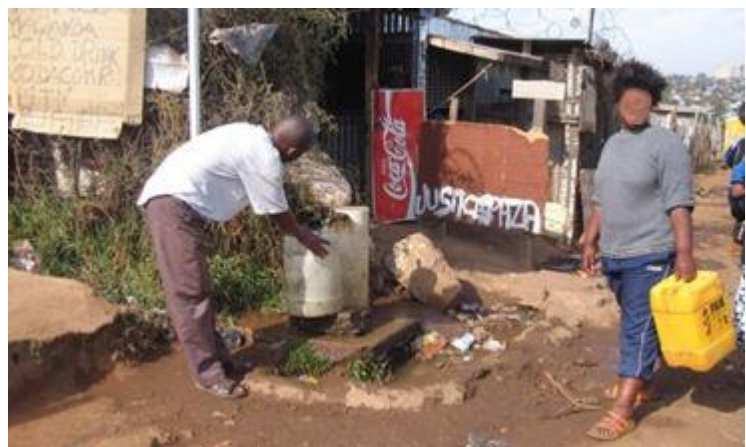
Figure 28: Collecting water from a communal street tap in Soweto, Johannesburg. Worn taps result in leaks and water wastage.
