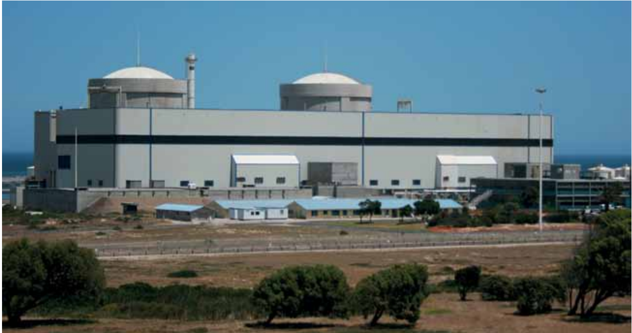
Figure 8: A nuclear power station
