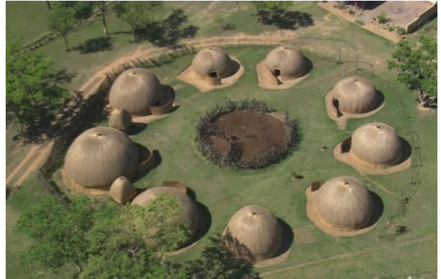
Inxuluma; grass; flat timber; logs floor-compressed cow dung; Kwazulu- Natal
