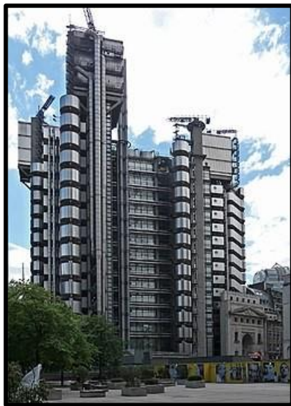
FIGURE 4b: Richard Rogers, Lloyds building , London, 1986.
