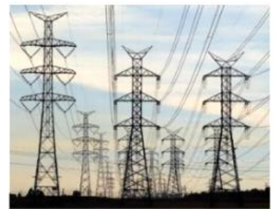
Figure 2 These pylons support the long transmission wires that carry electricity to all parts of our country—they are part of a nation-wide circuit called the national grid
