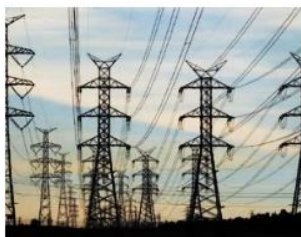
Figure 8 Tall pylons are the frame structures that support power lines
