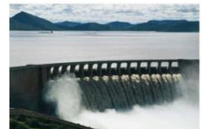
Figure 19 In this hydro-electric power station at Gariep in South Africa, water is dammed behind a wall and released through a turbine connected to a generator
