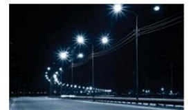
Figure 6 Electric circuit provides energy to street lights
