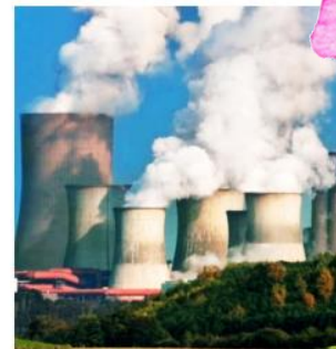
Figure 7 A coal-burning fire station
