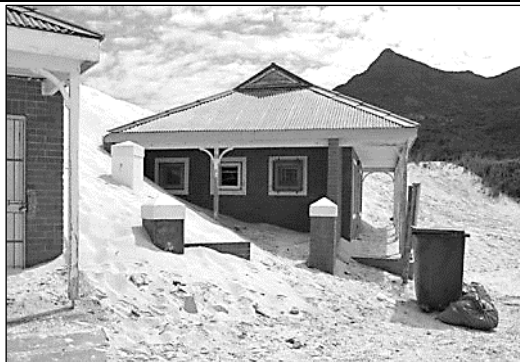
Image 1: Building covered in windblown sand
